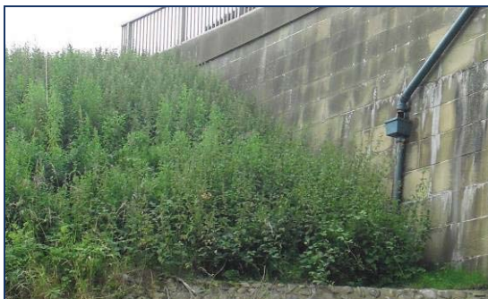
② Western embankment up onto A1 at Station Road
