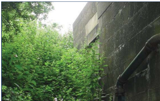
① Embankment up onto A1 at eastern side of bridge
