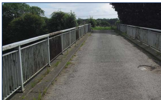
② Accommodation overbridge
