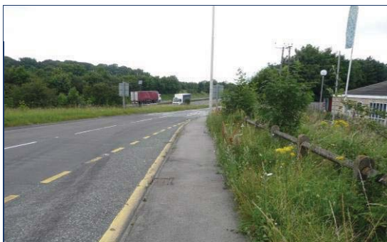
① Footway extending north on A1 southbound exit slip
