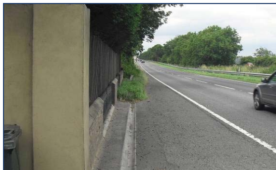
② Northbound carriageway north of access location
