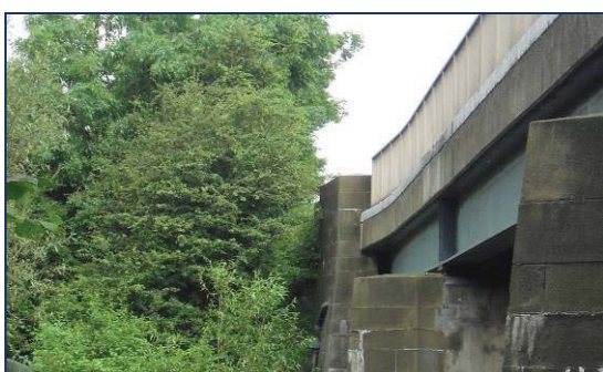
④ Bridge carrying A1 over River Swale (western face)
