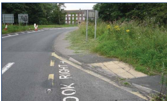
④ Restricted visibility at A1 northbound entry slip
