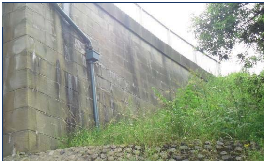
① Eastern embankment up onto A1 at Station Road
