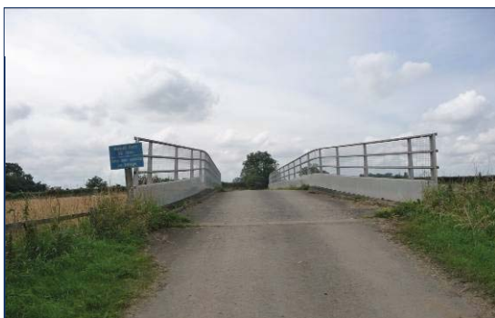
③ Accommodation overbridge at Manor House Farm
