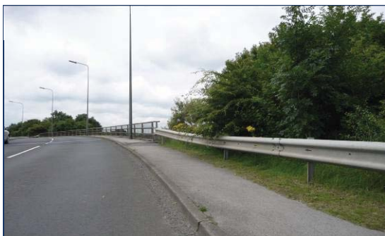
① Footway's eastern approach to overbridge
