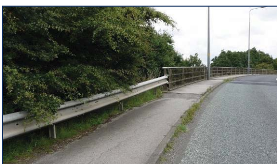
④ Footway's western approach to overbridge
