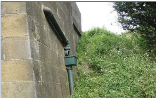
③ Embankment up onto A1 at eastern side of bridge
